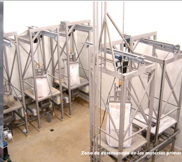
Sala de envasado FlowMatic
